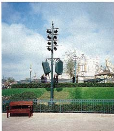
The walkway lampposts feature James Thomas Parcans and EAW speakers across the park, with 'intelligent control by Electrosonic (audio) and RV Electronique (light).
